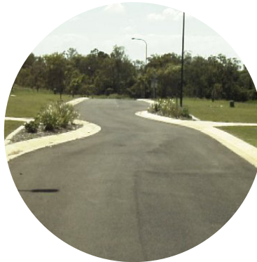
This chicane was designed to be part of a new development, though it is also feasible to retrofit a chicane. source: lgam.info
