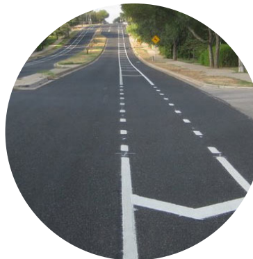
Buffered bike lane in Austin, TX, showing chevron buffer markings and dashed right turn transition source: NACTO
