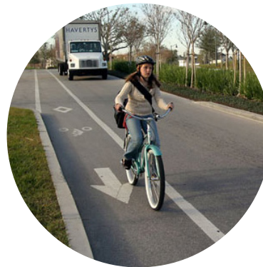
Conventional dedicated bike lane in Baldwin Park, CA, with appropriate roadway markings source: NACTO
