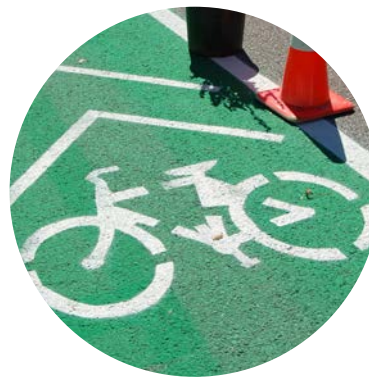
Temporary Shared Lane Markings (sharrows) were painted on the streets during the Street Smart demonstration weekend. source: CPEX
