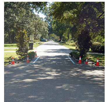
A traffic choker was installed on Richland Avenue to slow down speeding vehicles.
