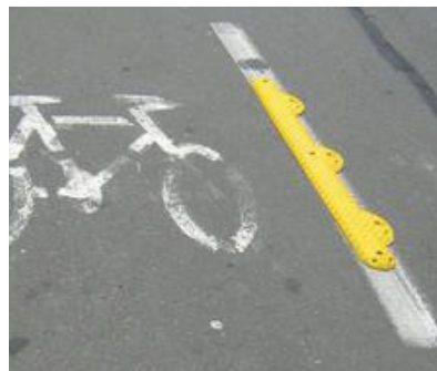
Low profile plastic lane separators add an additional layer of protection for cyclists without creating a dangerous obstacle for vehicles.
