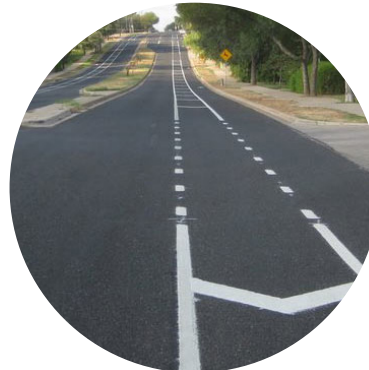
Buffered bike lane in Austin, TX, showing chevron buffer markings and dashed right turn transition
