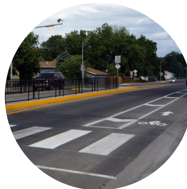
Buffered bike lane in conjunction with a high visibility crosswalk in Billings, MT
