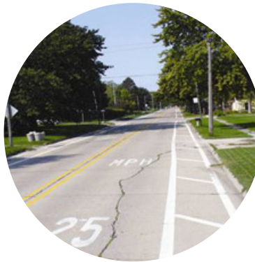
Extra wide streets can be narrowed through the addition of a striped buffer at the outside edge of the street. source: CPEX
