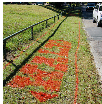
A “sidewalk” was installed to improve pedestrian connectivity between Capital Heights and Webb Park.
