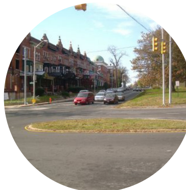
This example located in Baltimore, MD, shows an extended median that incorporates a U-turn area. source: NACTO
