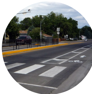
Buffered bike lane in conjunction with a high visibility crosswalk in Billings, MT source: NACTO
