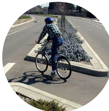
Bike refuges in medians provide bicyclists with a safe mid block crossing point. This example is located in Bellevue, WA. source: NACTO
