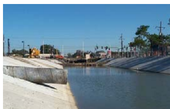
D-24 Typical concrete-lined channel with pipe outfall creates an ugly landscape, degrades water quality, and misses the opportunity to create a multiple-use corridor.
