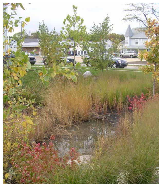
C-2 Bioswales, one of many natural ways of dispersing water runoff, contribute to sustainability. They also provide a public amenity for the neighborhood.
